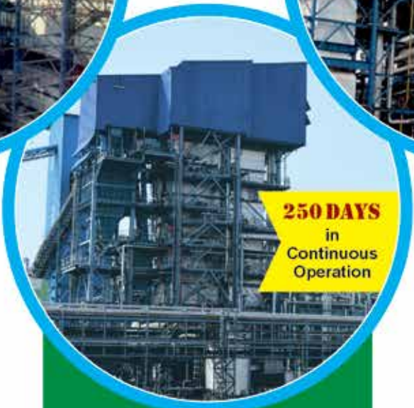
40 TPH Spent wash fired Travelling Grate Boiler at Dwarikesh Sugar, Bundki (U.P.)
